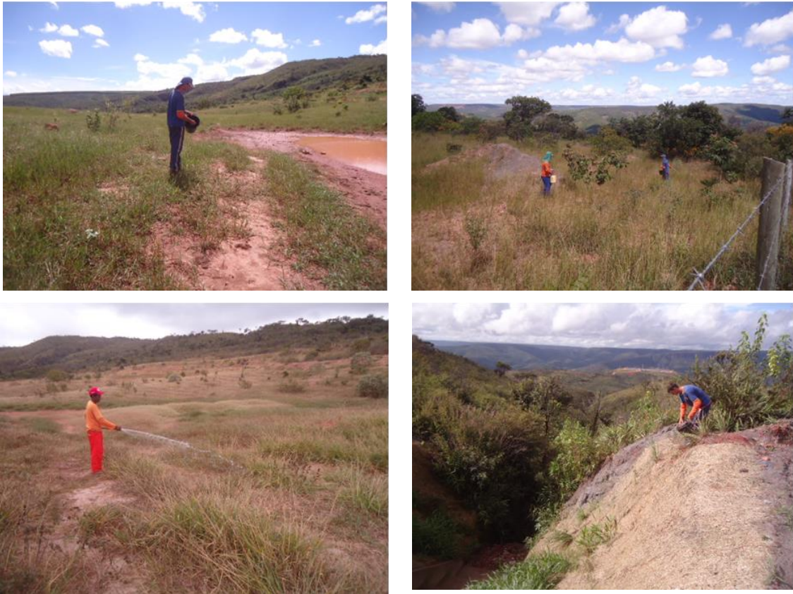
Figure 33. Maintenance activities in degraded areas recovery plan for Irapé HPP
