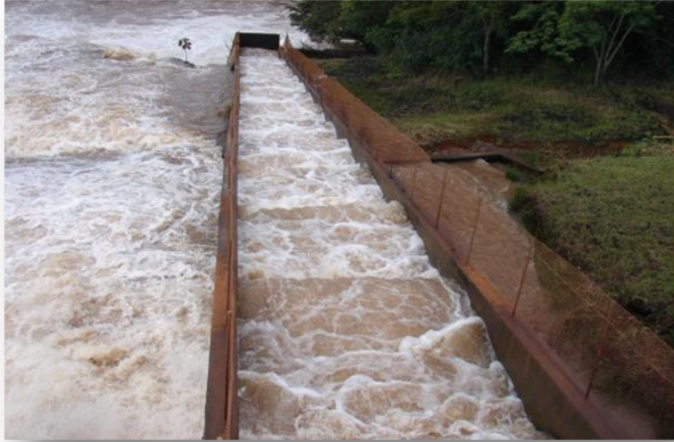
Figure 20. Fish ladder system at the Salta Moraes Hydroelectric Power Plant
