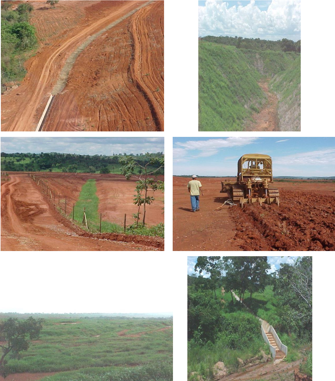
Figure 32. Operations for deployment of the degraded areas recovery plan (PRAD) – Emborcação HPP
