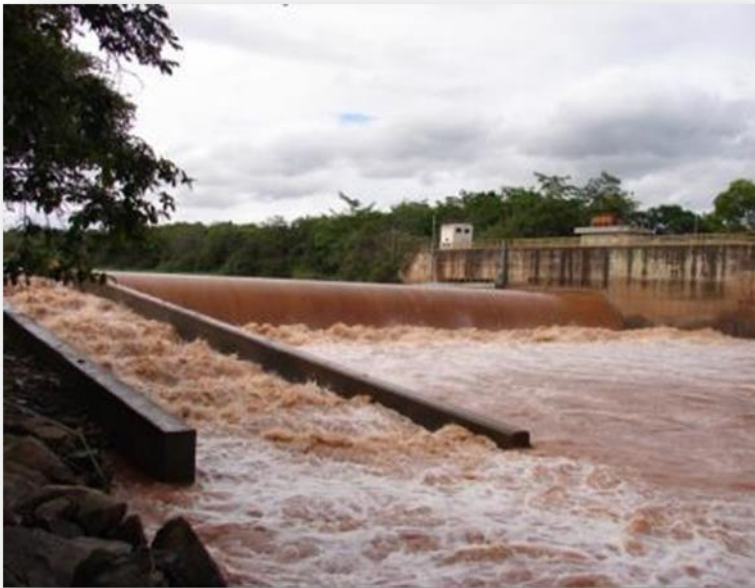
Figure 21. Fish ladder system at the Igarapé Thermal Power Plant
