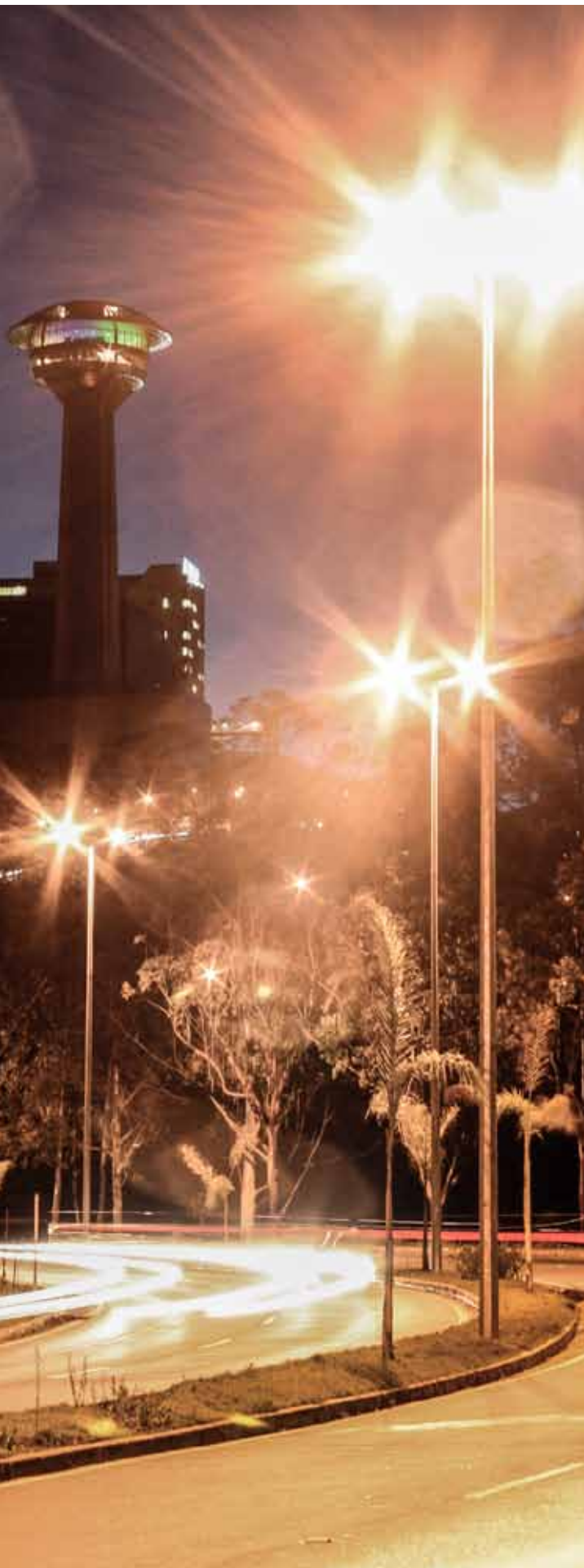
PUBLIC LIGHTING – BELO HORIZONTE
