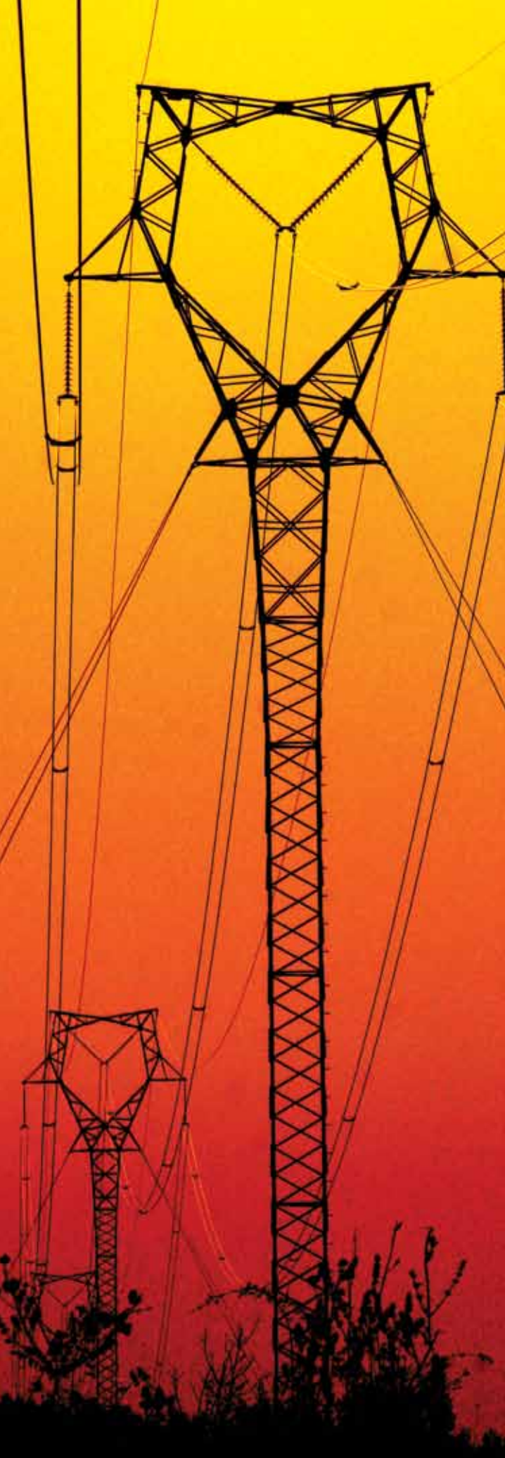
TRANSMISSION LINES – IRAPÉ
