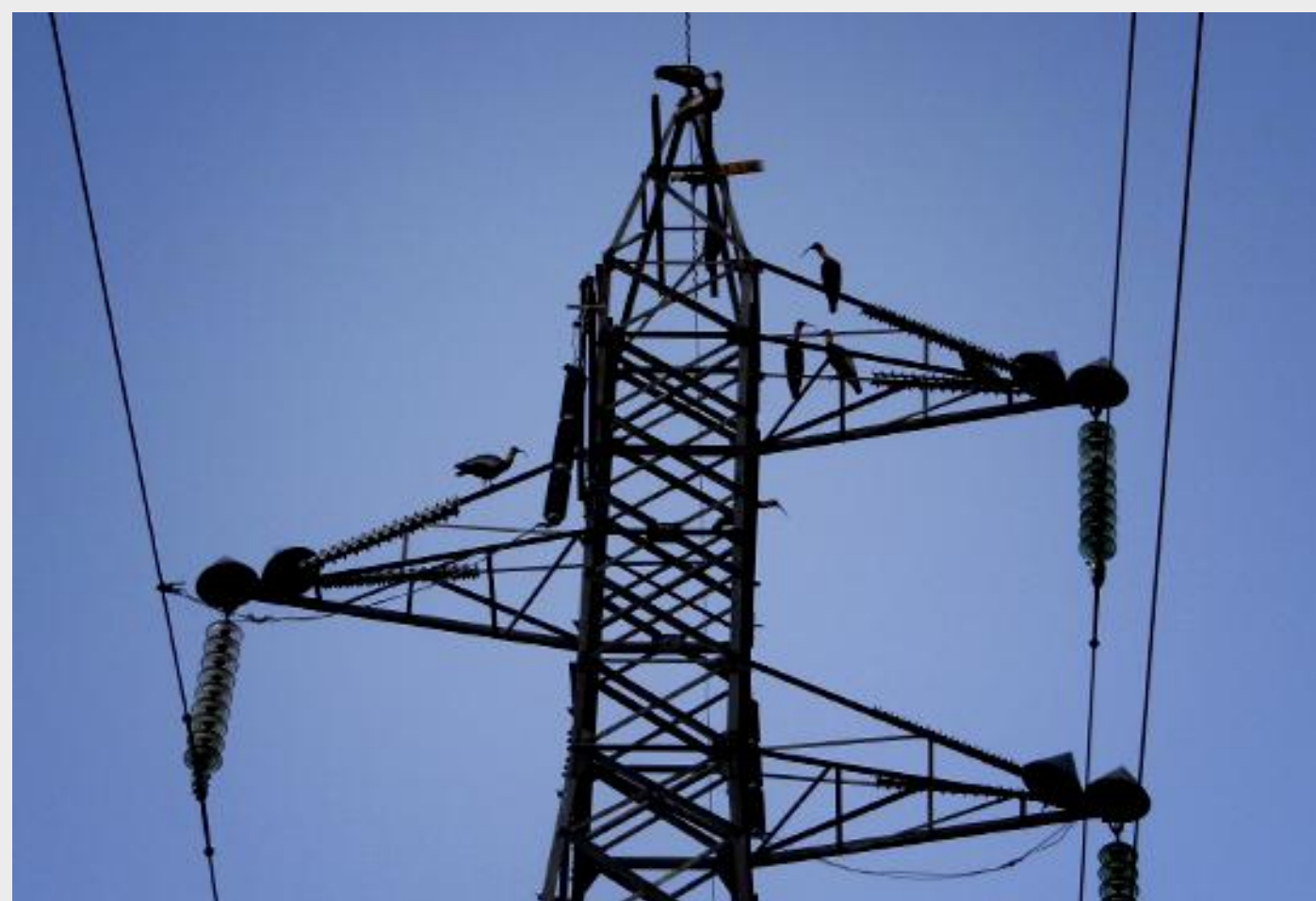
Cone to discourage bird perch
