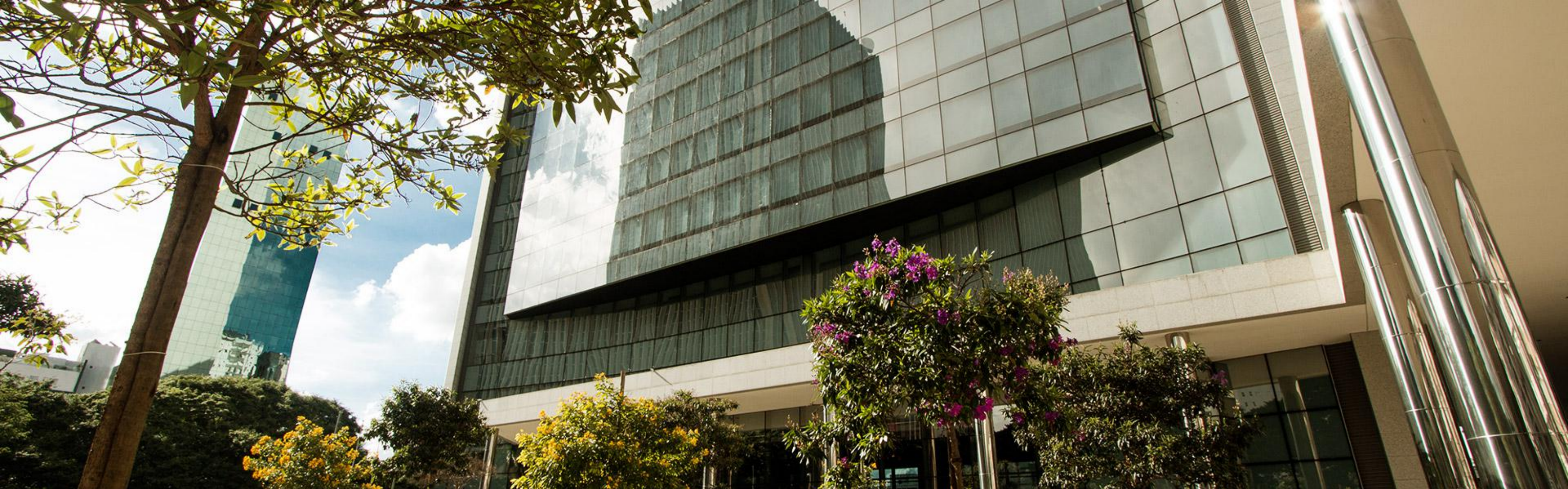
Aureliano Chaves Building and Júlio Soares Building, headquarters of Cemig.
