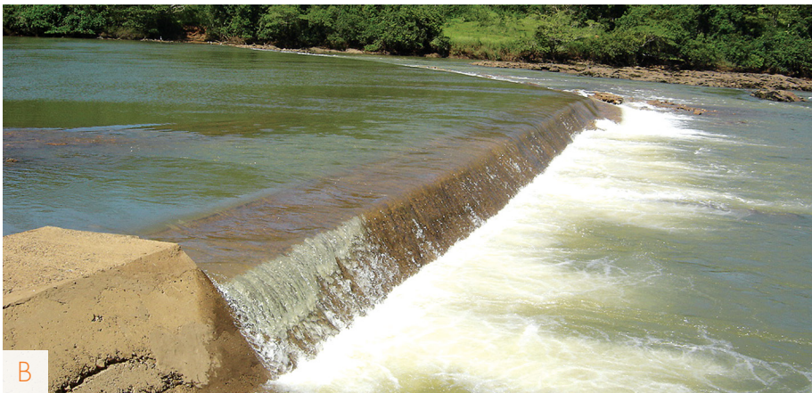
FIGURE 3 – The reduced outflow stretch of the Amador Aguiar I Dam before (A) and after (B) the regularization to eliminate the various fish entrapment spots. Photos: Lazaro Carlos de Freitas.
