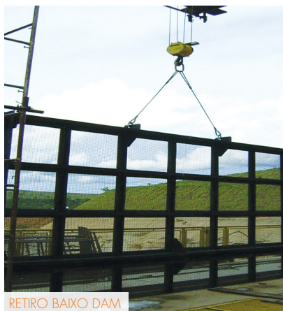
FIGURE 1 – Fish screen system at hydropower plants of Cemig Group.
