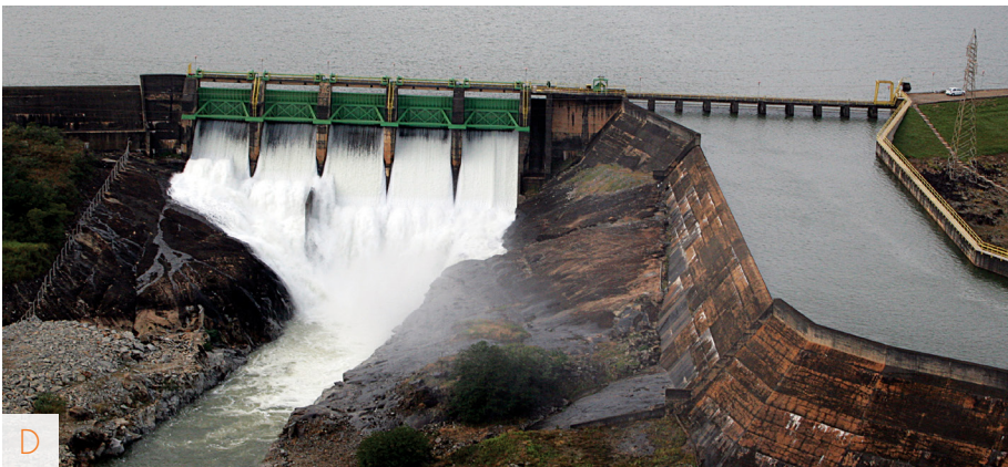
FIGURE 2 – The spillway dissipation basins of Jaguara (A) and Itutinga (B) dams, with people catching fish after spillway closure. Spillway dissipation basin after work to remove fish entrapment spots at Jaguara (C) and Itutinga (D) dams.
