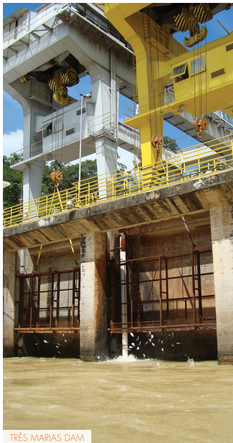
FIGURE 1 – Fish screen system at hydropower plants of Cemig Group.
