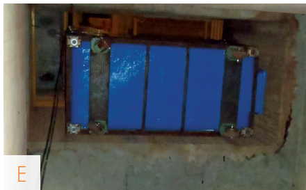
FIGURE 7 – Platform mounted inside the draft tube of São Simão Dam (A). Fish transport box positioned at the exit of the draft tube hatch (B). Ramp set at the opening of the transport box for transferring fish recovered from the draft tube (C). Transport box being hoisted through the block outs of the plant (D and E). Transport box being loaded on a truck that will take the recovered fish to the release area (F). Photos: Átila Rodrigues (A) and Alexandre Peressin (B to F).
